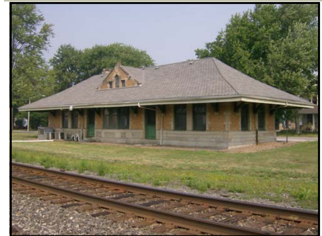
Stryker's former Lake Shore & Michigan Southern/New York Central Railroad passenger station, listed on the National Register of Historic Places, symbolizes the community's rich railroad heritage
