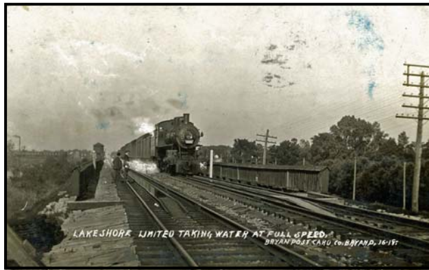
A steam locomotive scoops up water "on the fly" at the Tiffin River track pans in Stryker
