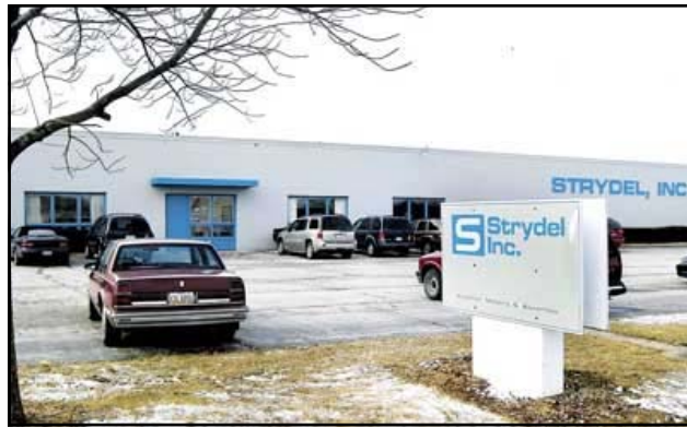
The Strydel, Inc., facility located at 201 Ellis Street in Stryker
